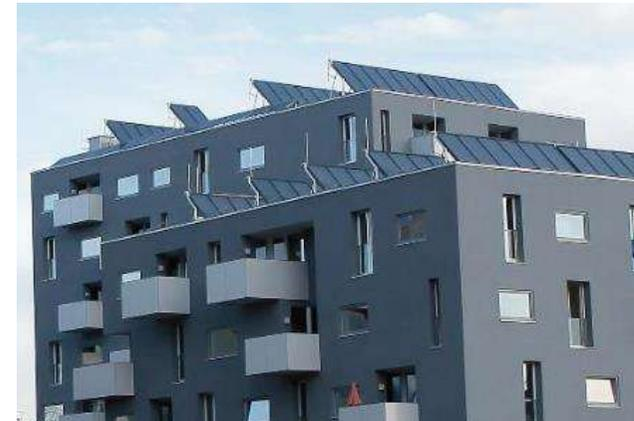
**1.500 kW heat (2.150 m<sup>2</sup> collector)**
