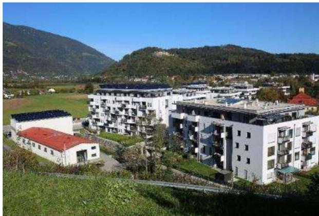
**680 kW heat (970 m<sup>2</sup> collector)**
