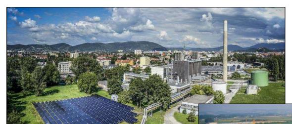
Solar process heat for industrial purpose 1.400 m<sup>2</sup> (1 MW)
